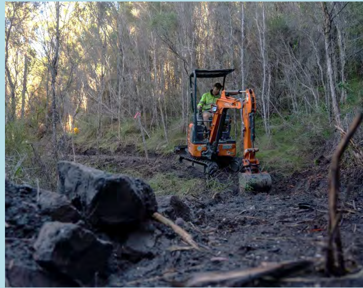
Wild Mersey Mountain Bike Trails being constructed.
