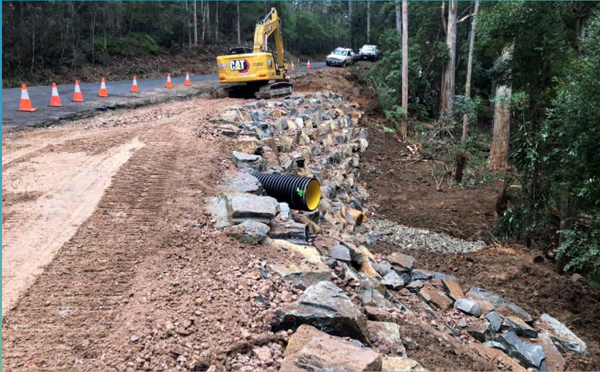
Road land slip repair works
