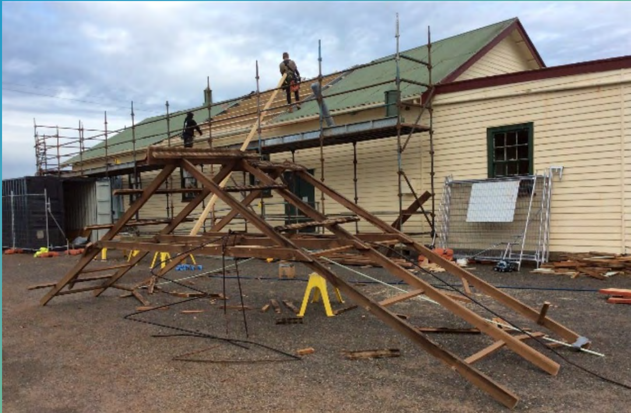
Barrington Hall being re-roofed
