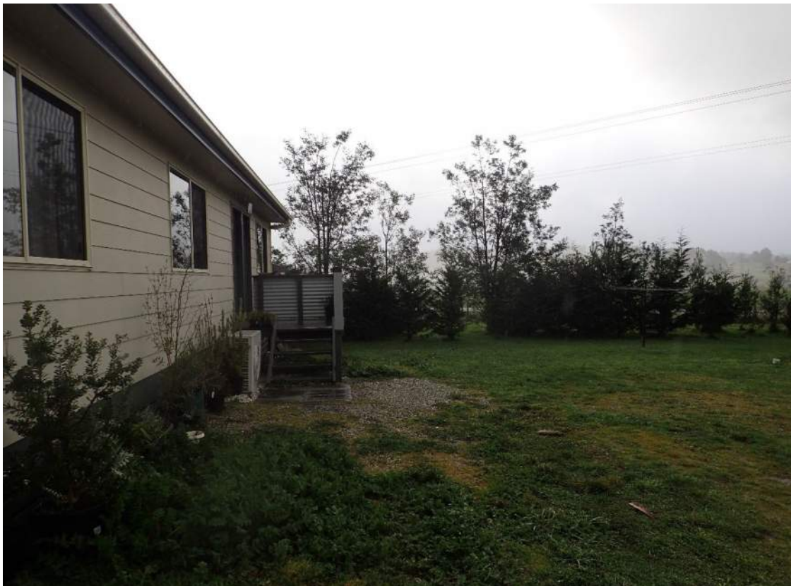
NORTH WEST View showing the elevation of the new proposed deck. The grassland vegetation is consistent to the boundary.
