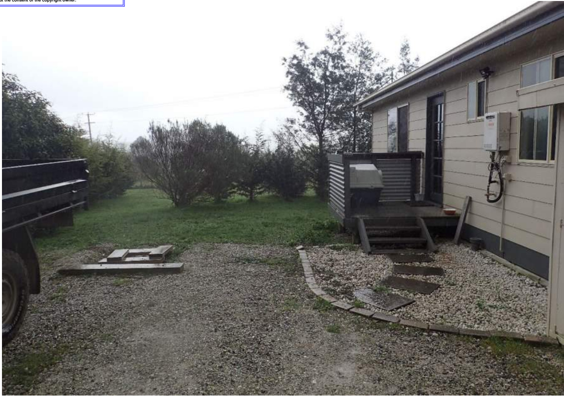
NORTH WEST View from the area of the new shed & walkway.
